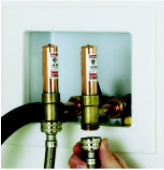
Washing Machine Install between laundry supply valves and hoses
